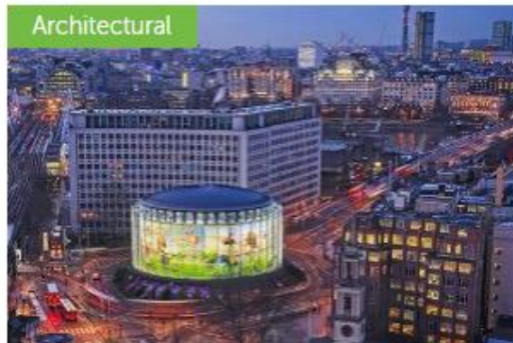
IMAX Waterloo, London > Constant voltage LED drivers and DMX control
